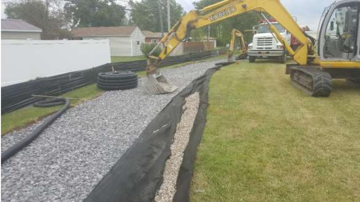
Figure 3 Typical porous path section including geotextile, underdrain and BUD Corian underdrain stone
