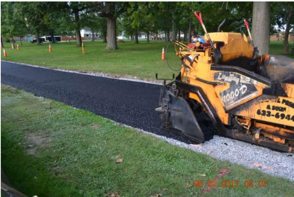
Figure 4 Contractor placing porous asphalt over choker course
